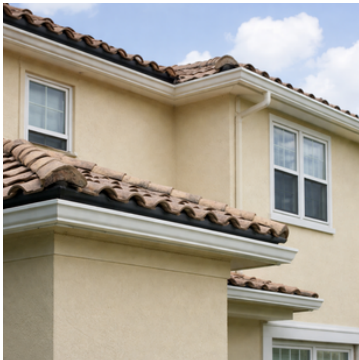
Exterior condition- no issues observed
