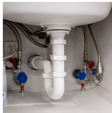
Plumbing inspection - no leaks detected
